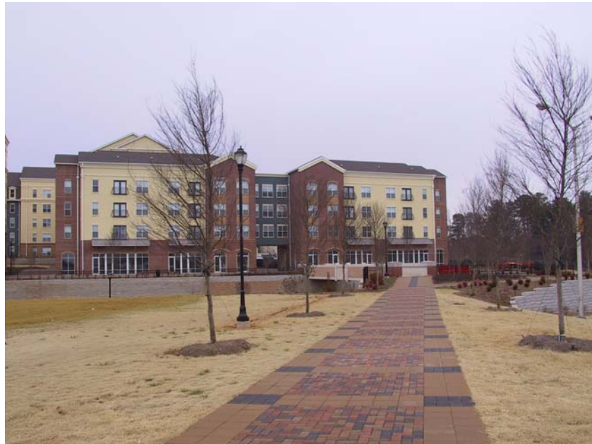
The existing North Campus Walk is a prime segment of the north-south circulation “spine”, and is enhanced by wide pathways of distinctive paving.
