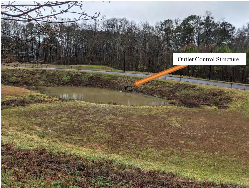
Photo 10: View of large stormwater pond and outlet control structure (OCS2539) near Hornet Village that discharges to SW-M08.
