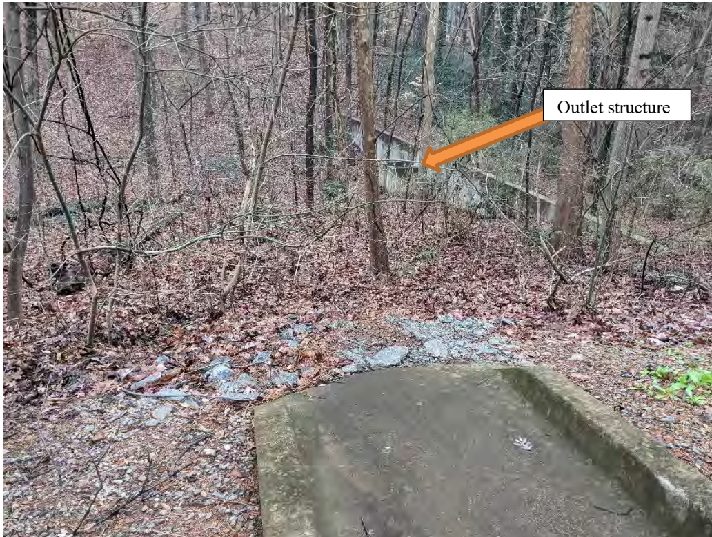
Photo 5: View of SW-K05, located near the Technology Services building.
