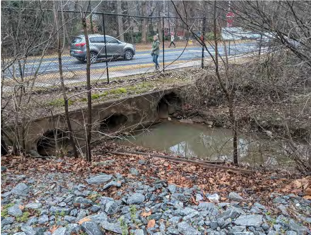
Photo 3: View of SW-K03, located north of West Parking Lot.
