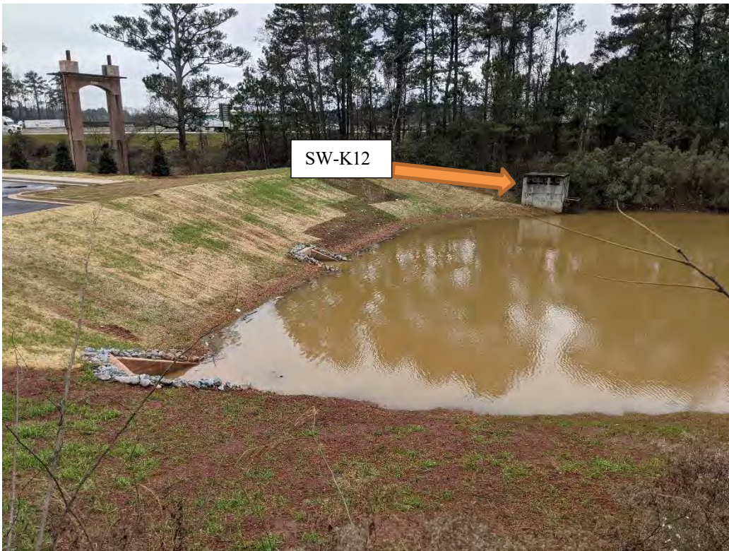
Photo 14: View of SW-K12 (outlet control structure) and southern portion of stormwater pond located near the Surplus building/ Shuttle Lot.
