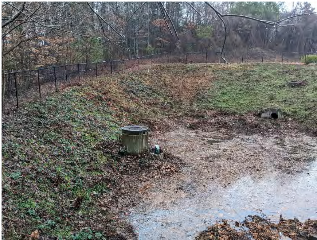
Photo 4: View of pond and outlet control structure (OCS2941) directly upstream of SW-M03.
