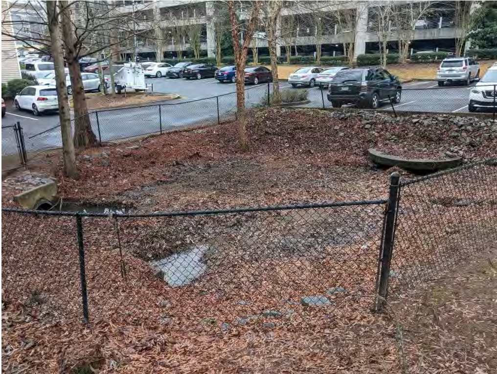
Photo 7: View of detention basin near the North Parking Deck which discharges to SW-K06.
