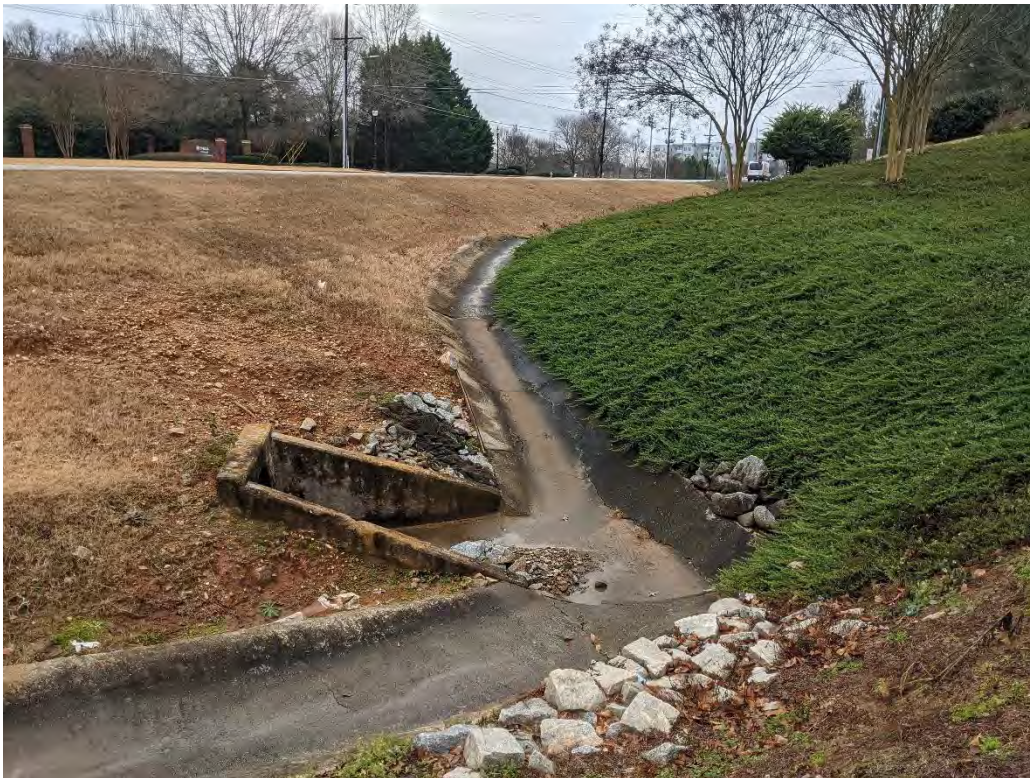
Photo 12: View of outfall SW-K10 located along Busbee Drive near KSU Center.
