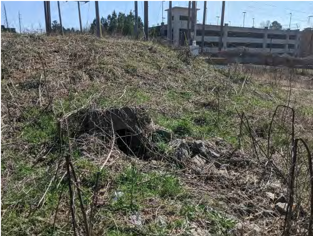
Photo 24: View of SW-M21 (headwall) located near Facilities building.
