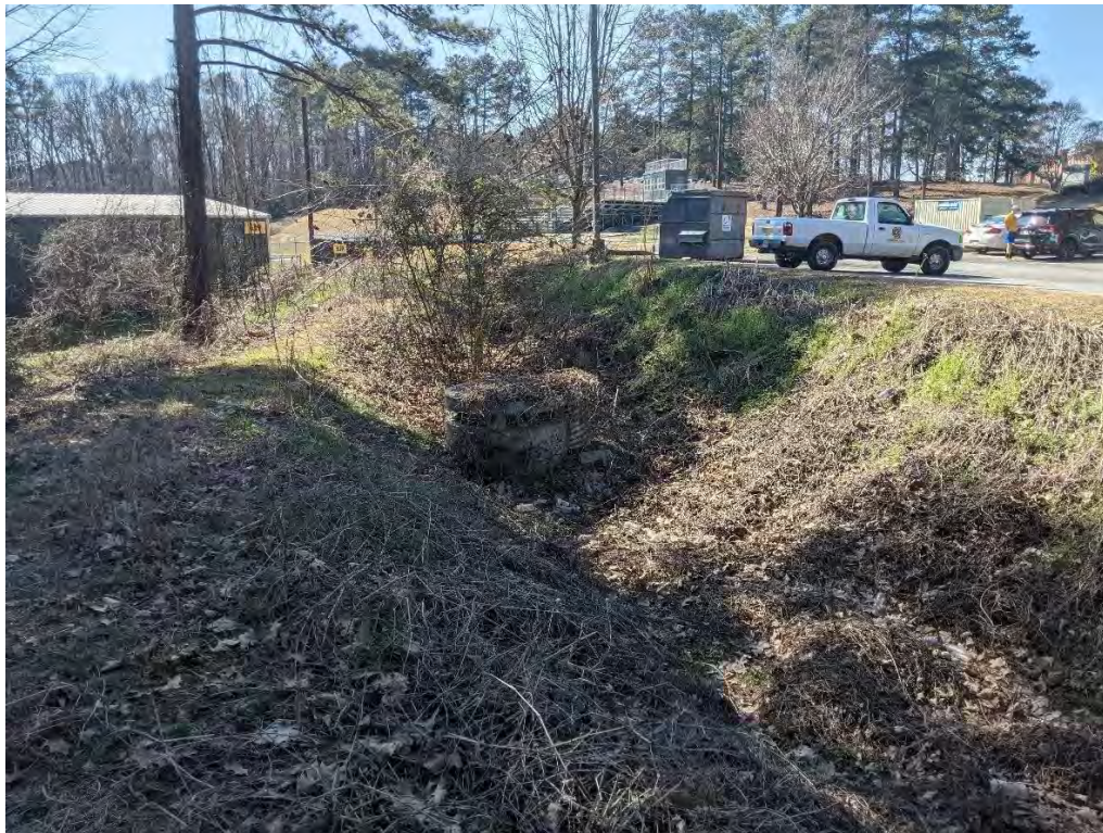
Photo 16: View of detention pond and outlet control structure (OCS19) discharging to SW-M13.
