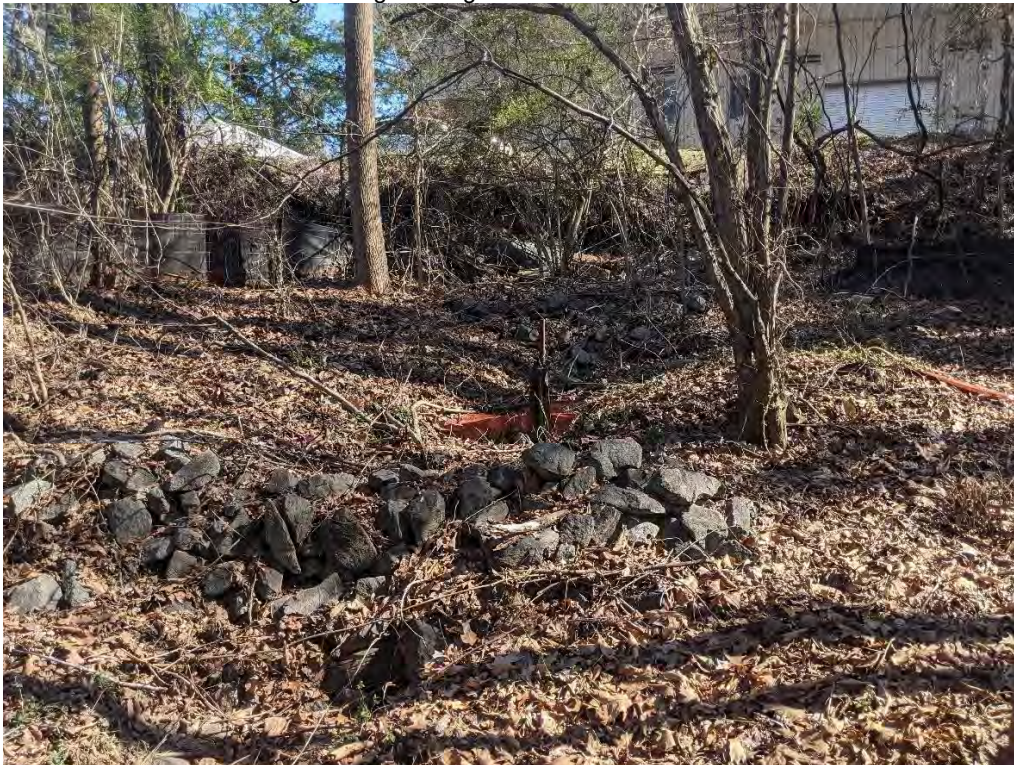
Photo 12: View of SW-M10 (for sheet flow) off the northeast corner of the Student Competition Team Building.
