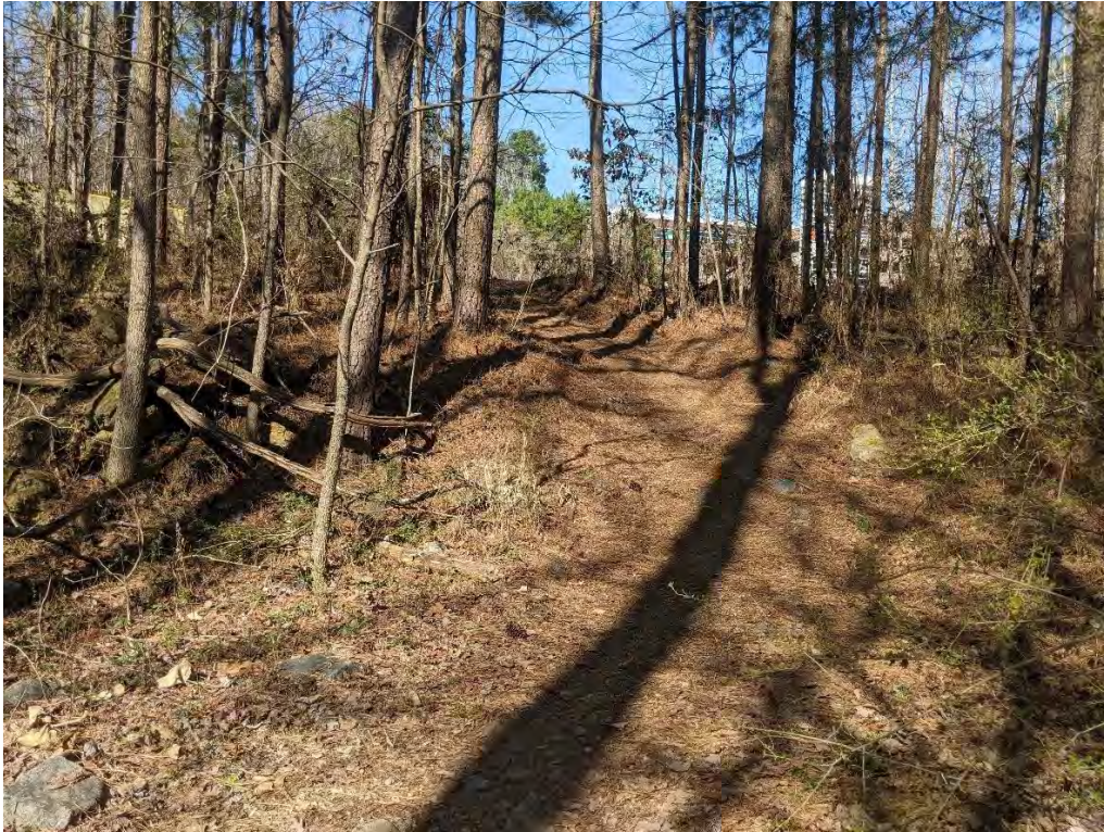
Photo 5: View of SW-M04 located at the southern corner of Polytechnic Lane and Alumni Drive, which discharges sheet flow from Polytechnic Lane.
