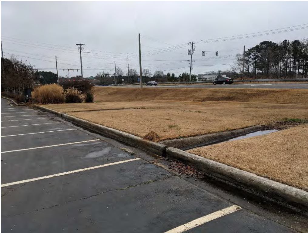
Photo 13: View of outfall SW-K11 located along Busbee Drive near former hotel.
