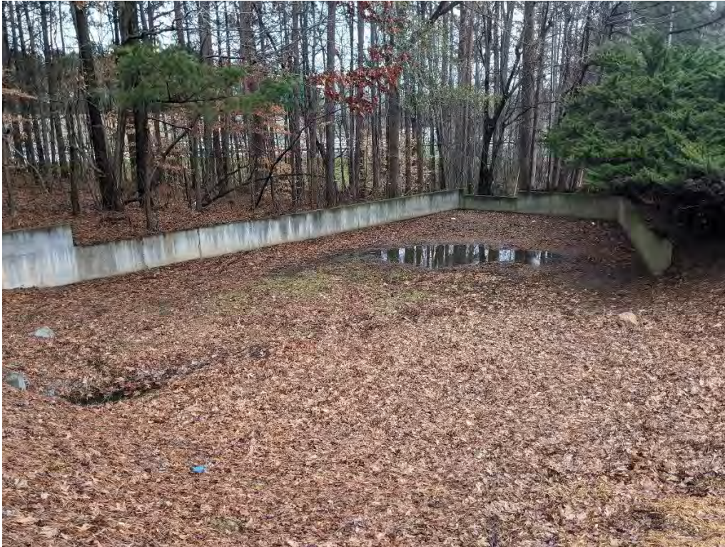
Photo 9: View detention area and outfall SW-K07 located south of KSU Place Apartments.
