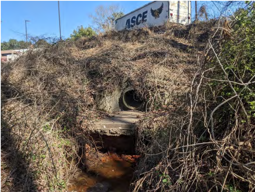
Photo 11: View of SW-M09 located off northwest corner of lot P23 near the Civil and Environmental Engineering building.
