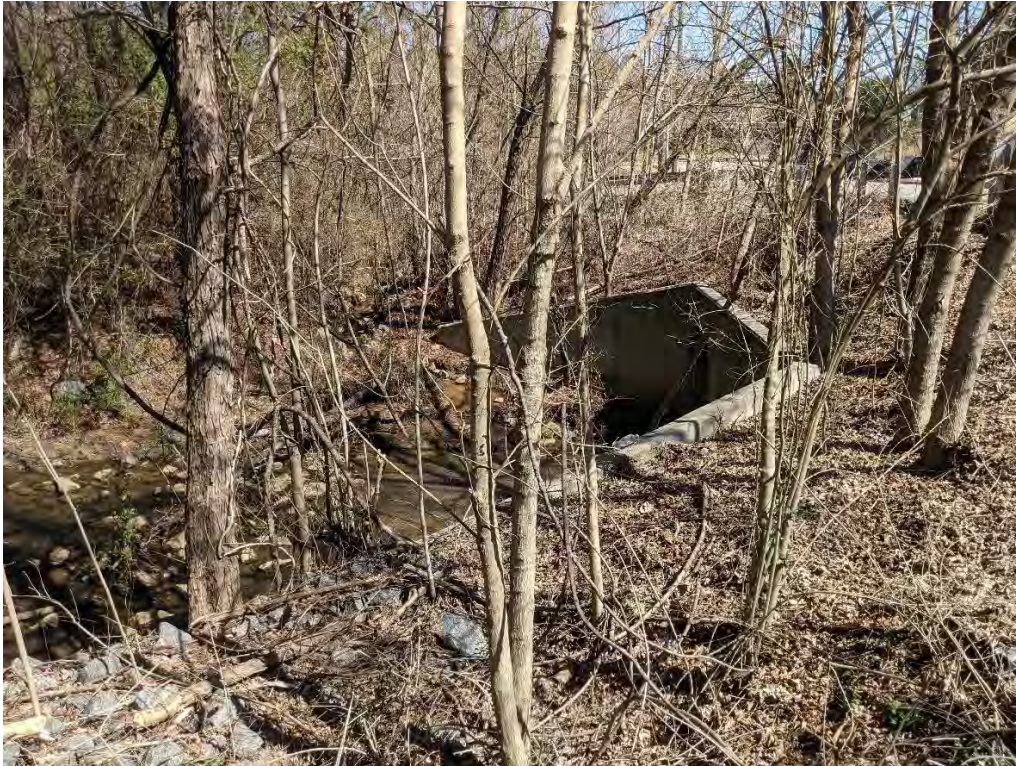
Photo 21: View of SW-K13, along Big Shanty Road, which serves as the main discharge point for stadium area.
