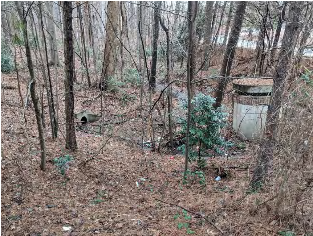
Photo 22: View of Outfall SW-K14 (outlet control structure) in detention pond located on southeast portion of Town Point.
