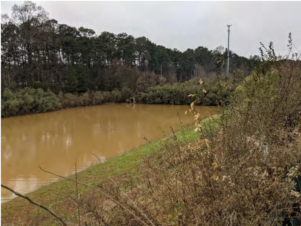
Photo 15: View of headwalls located on northern portion of stormwater pond near the Surplus building/ Shuttle Lot.
